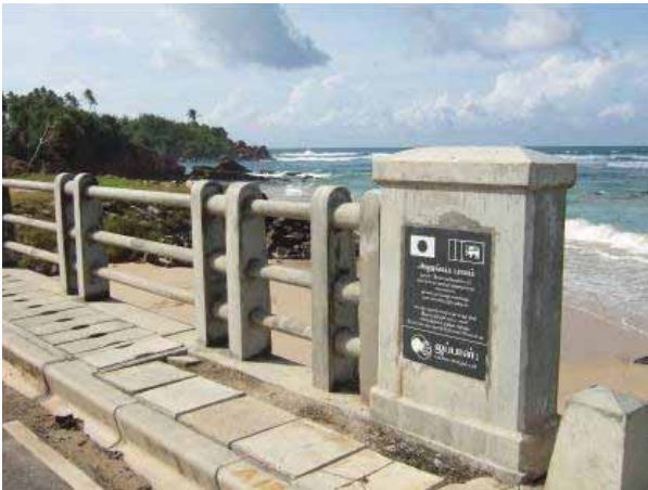
Ahangama Bridge [Non-Project Grant Aid]
