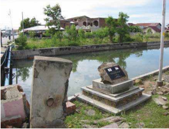
Bank Strengthening Works [Non-Project Grant Aid]
