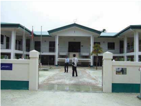
Administrative Office/ Multi-Purpose Building in Gan Island, Laamu Atoll [Non-Project Grant Aid]
