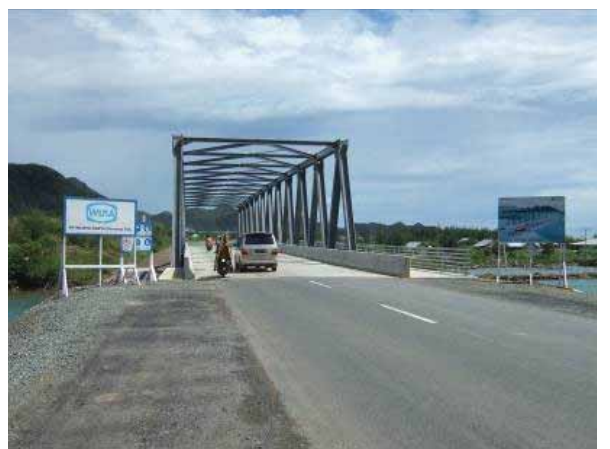
USAID's West Coast Road Construction Project (Banda Aceh – Chalang)
