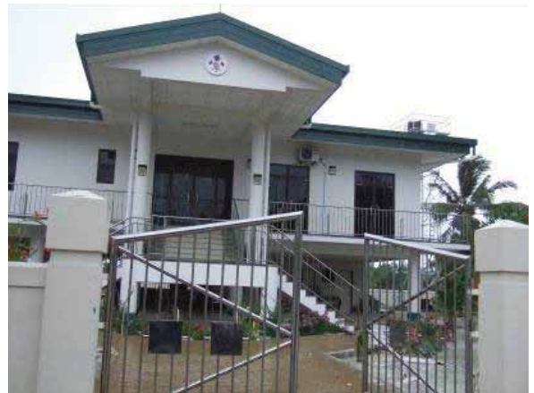
Administrative Office in Fonadhoo Island, Laamu Atoll [Non-Project Grant Aid]
