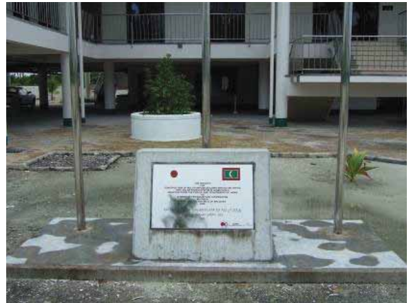
Administrative Office/ Multi-Purpose Building in Gan Island, Laamu Atoll [Non-Project Grant Aid]
