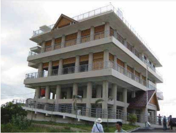
Evacuation tower/Community Hall [Non-Project Grant Aid]
